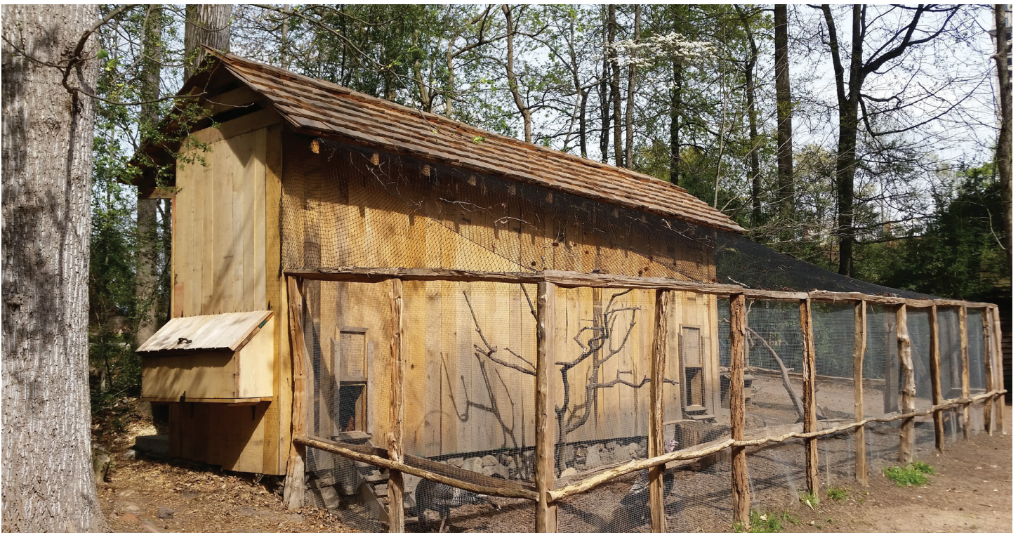
A reconstruction of what a mid-nineteenth century chicken coop may have looked like in Georgia. The coop is made from oak with a cedar shake roof and locust poles to frame the enclosed run. The bird netting and hardware cloth is a necessary adaptation to protect from hawks and other predators. Smith Family Farm. Photograph by Sarah Roberts.
